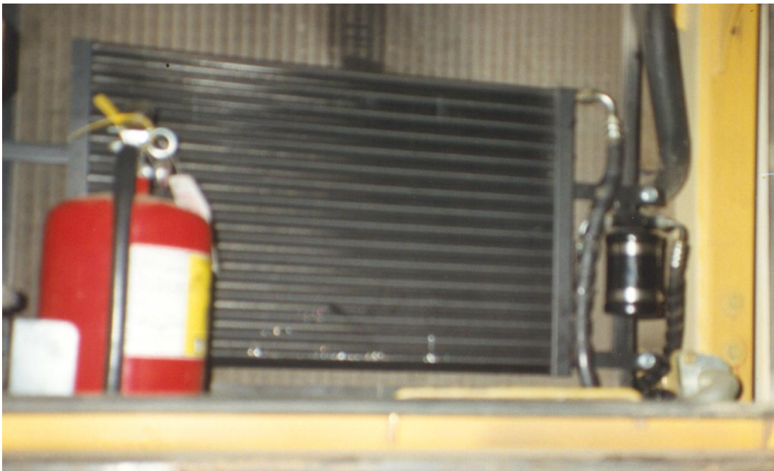
Condenser mounted in location.
